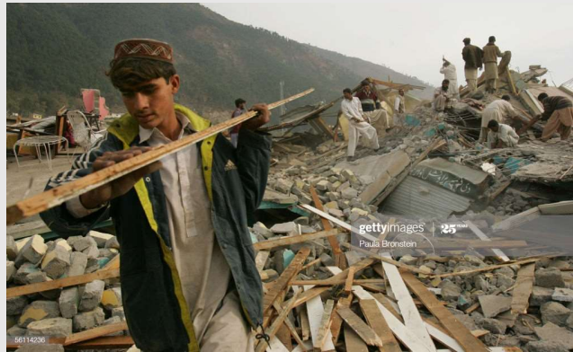
a worker helps to clear the debris.
