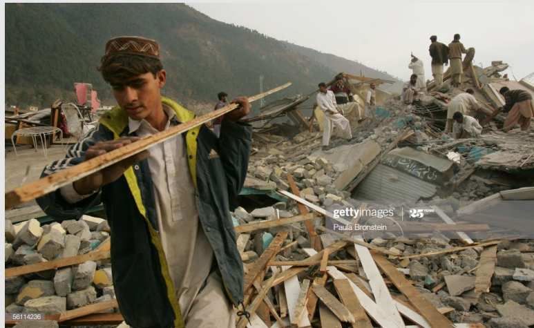
a worker helps to clear the debris.
