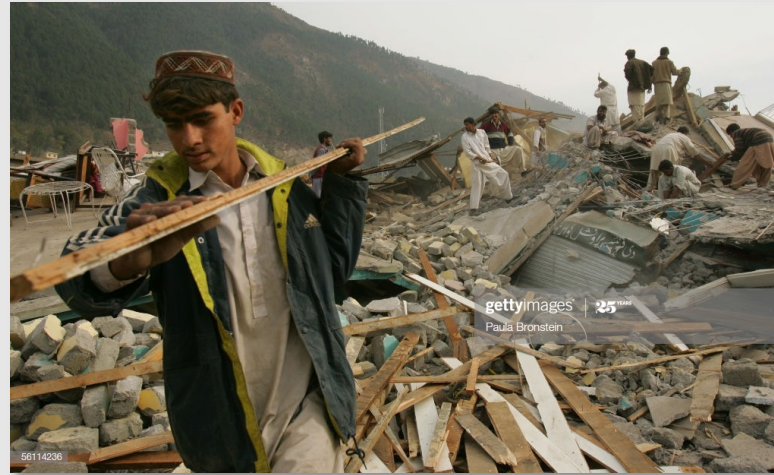
a worker helps to clear the debris.
