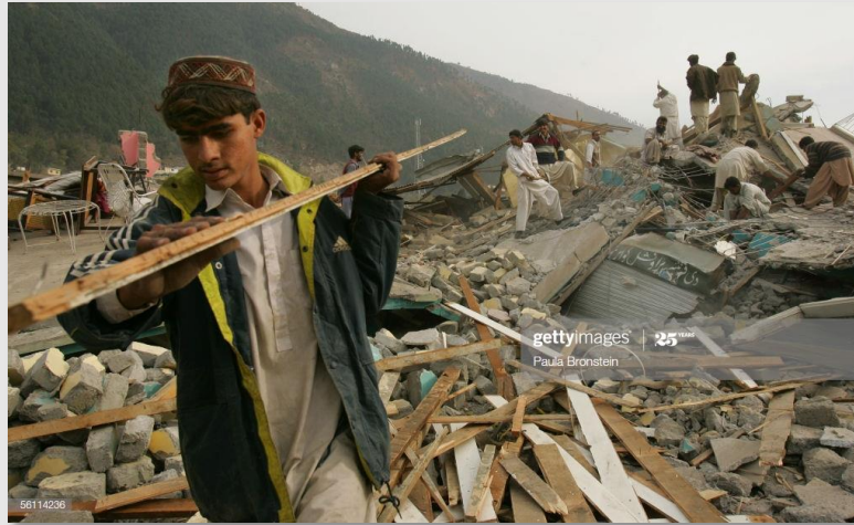
a worker helps to clear the debris.
